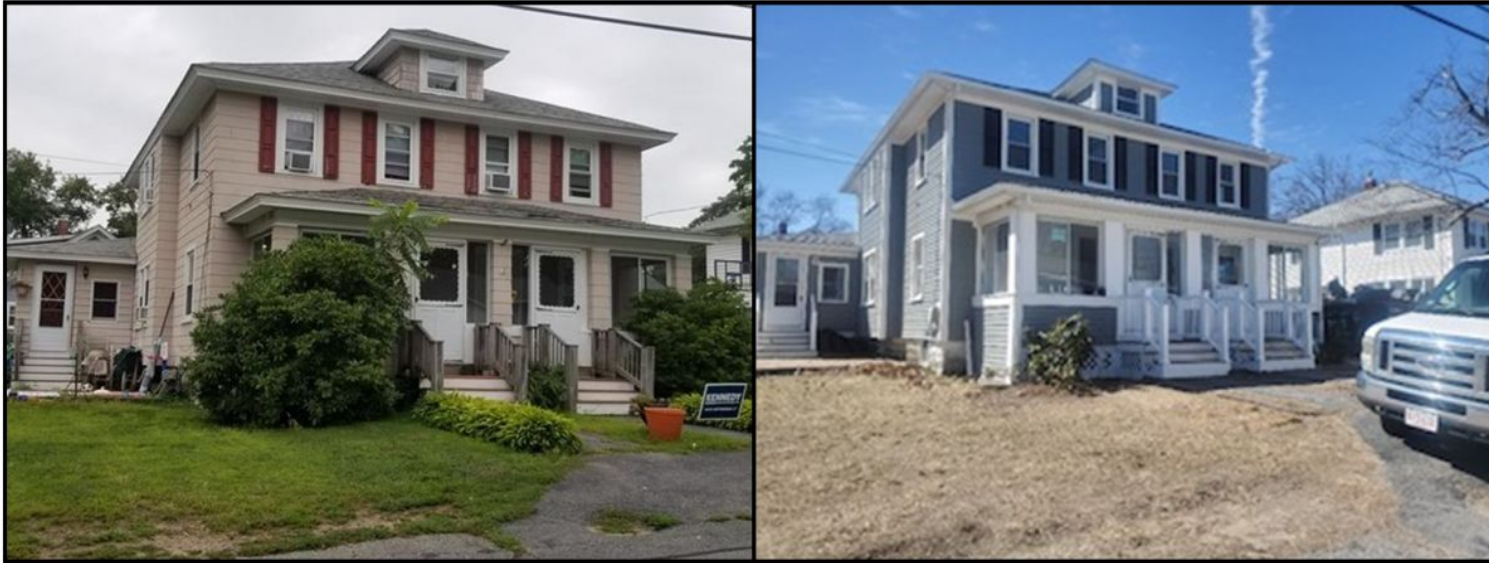
Image: A duplex purchased and renovated by the Billerica Affordable Housing Trust and Billerica Housing Authority (via communitypreservation.org )
