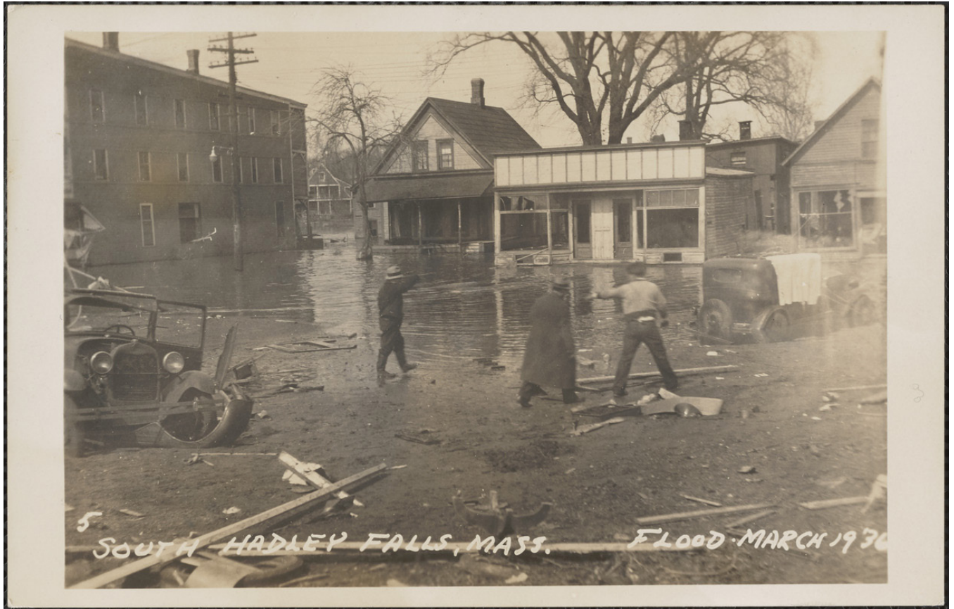
Figure 32: A photograph of flooding in South Hadley Falls, 1936
